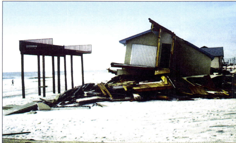
Damage from Hurricane Opal in Florida. This deck was designed to meet State of Florida Coastal Construction Control Line (CCCL) requirements. The house predated the CCCL and did not meet the requirements.
