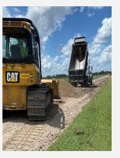
Precinct 2 Road and Bridge has been busy improving the road leading to the Angleton Soccer Complex. Through an interlocal with the City of Angleton, crews are recycling the old asphalt into base material, adding crushed concrete and restabilizing cement for a stronger base before paving with asphalt.
