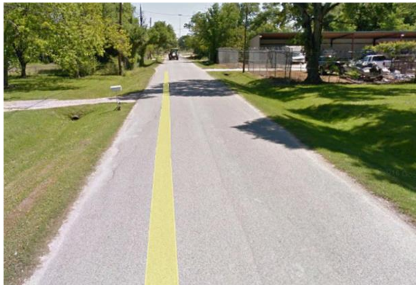
Figure 2-14 Roadside Ditch (R) Example
